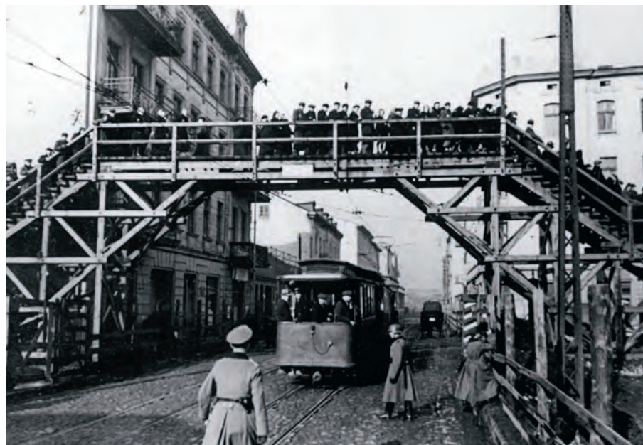
A pedestrian bridge over an “Aryan” street in the Łódź ghetto in Poland. Jews in the ghettos were strictly segregated from the rest of the world. In larger ghettos with more than one area, such bridges were sometimes built to connect Jewish sections divided by “Aryan” thoroughfares. The crowding on the bridge reflects the living conditions in the ghetto: a very large number of people existing in a very small area.
